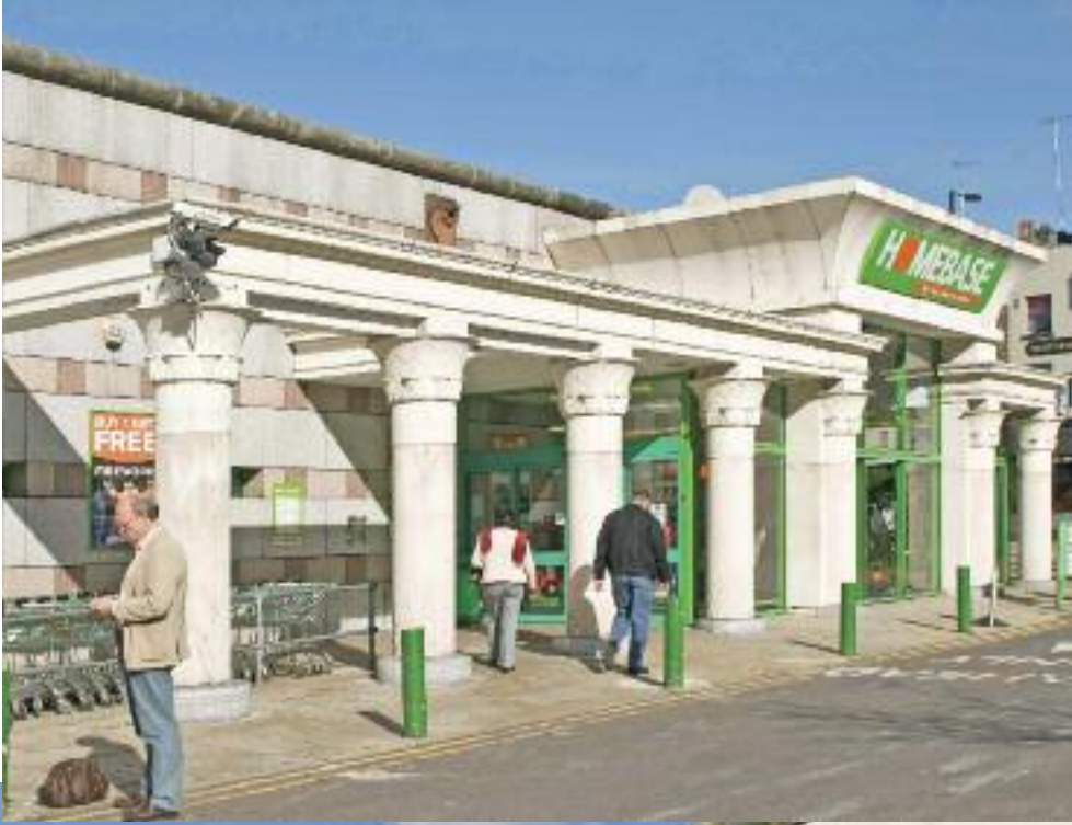
Homebase DIY superstore in London is the most recent Egyptian-style building in England (completed in 1988), with composite columns & entablature marking the entrance (left), & a sunk-relief frieze parade of ancient Egyptian deities on the structure's exterior wall (below).
