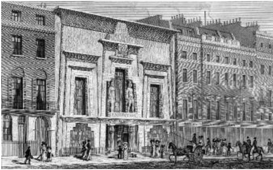
Left, The first example of an Egyptian-style façade on a major public building in England, designed by Peter Frederick Robinson, was the 1811-1812 Egyptian Hall in Piccadilly, built to house the London Museum of William Bullock. XA00143
